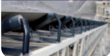
Figure 3: high levels of roll drag associated with idler sets increase energy consumption
